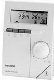
Room unit QAW70 with room temperature detector, time switch, setpoint adjustment, and room temperature readjustment (setting knob)
